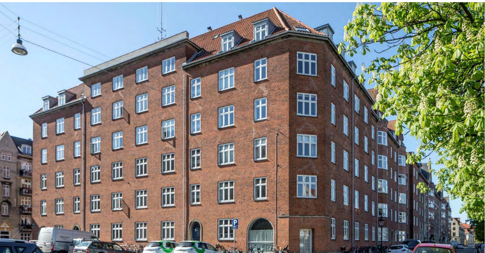
Overgaden Oven Vandet, Christianshavn, Copenhagen
