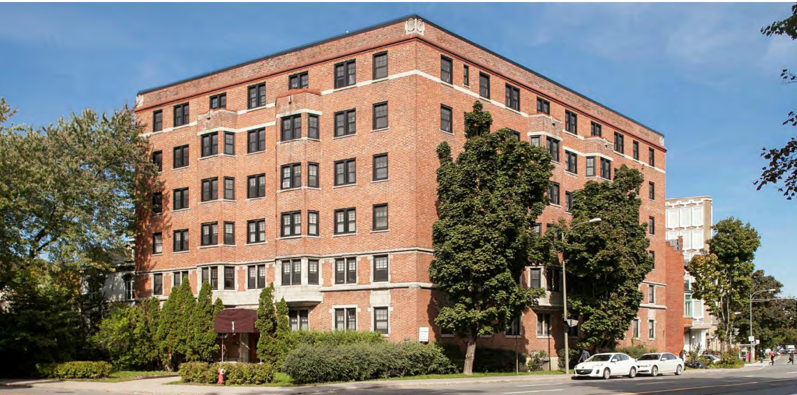
1 Rosemont Avenue, Westmount, Montreal
